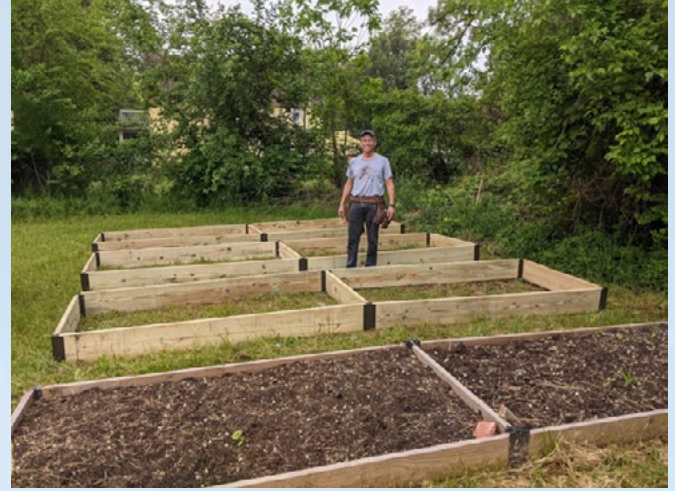
Raised garden beds under construction, May 8, 2024. Trinity Farm Volunteer Paul Hergasell checks on progress.
